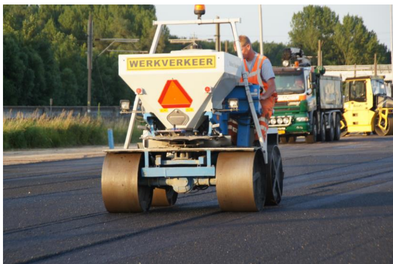
Figure 7: Developed sanding equipment for the OPA8.
