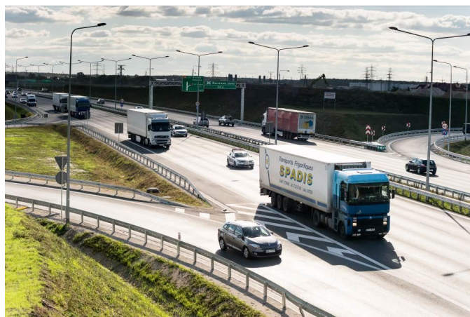
Figure 10: Expressway S8 between Opacz and Paszków with perpetual pavement opened to traffic in July 2015 – 5 months before schedule
