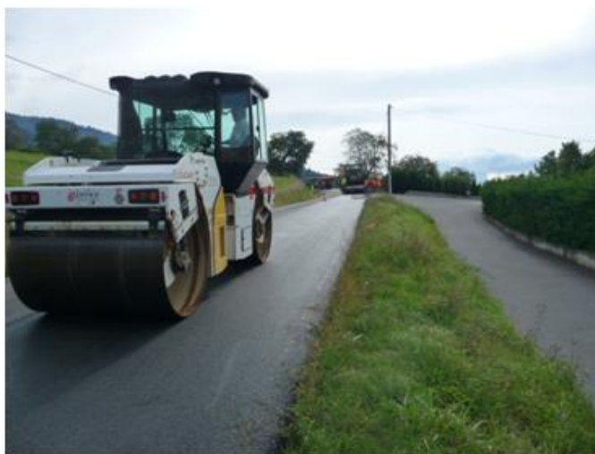
Figure 4: WMA application in Lucinges in september 2013
