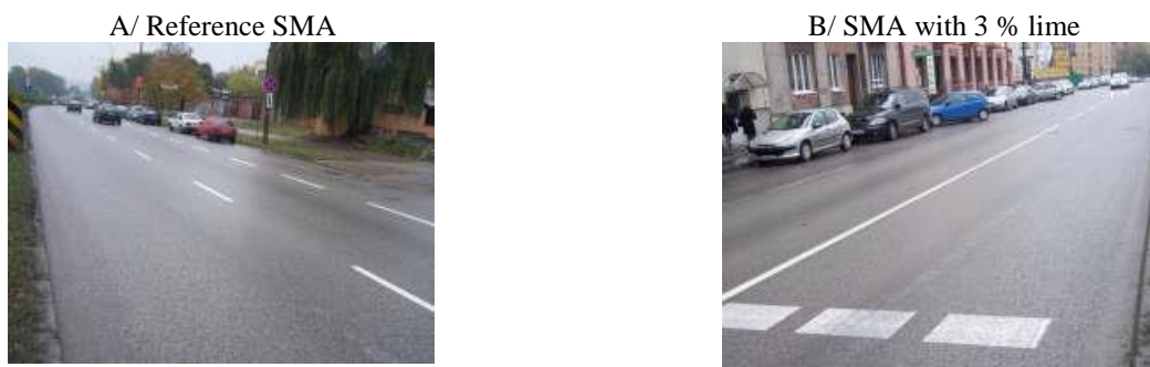
Figure 4: View of the reference section (A) and the section with lime (B) on Zelazna street after 11 years. From [17].
