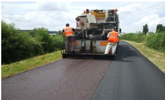
Photo 9: View of the jobsite during application
