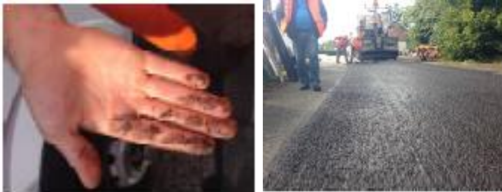
Photo 5 and 6: Unbroken emulsion on jobsite
