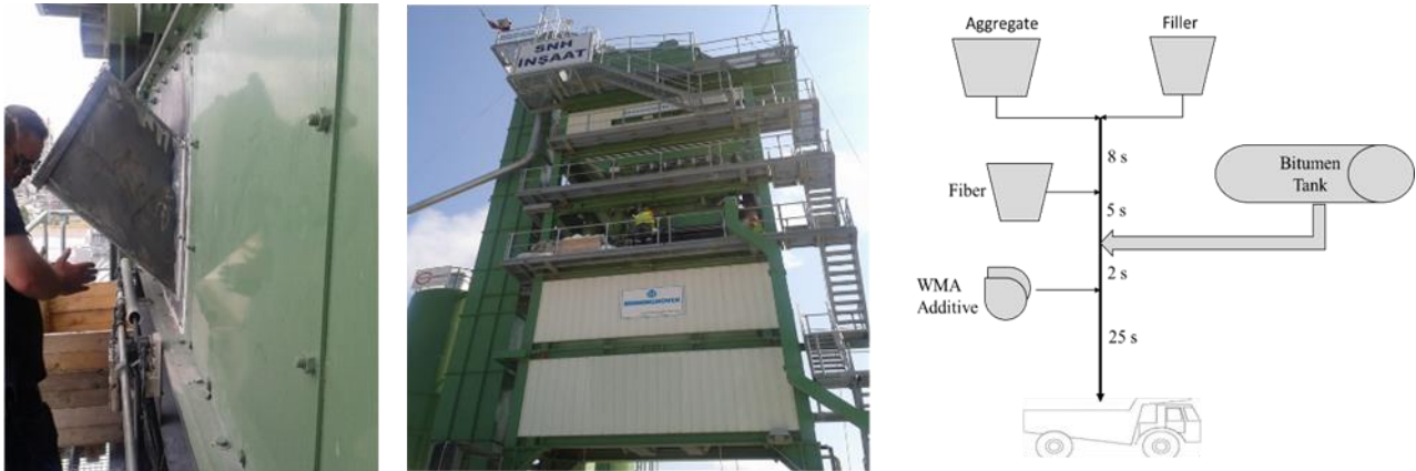
Figure 11: Pictures of asphalt plant showing feeding system and time synchronization.
