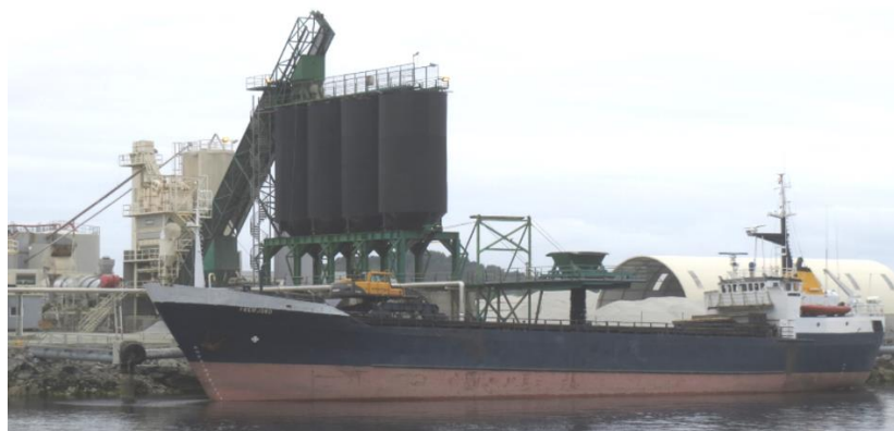
Figure 9: Asphalt plant and loading of boat (Photo: Bjørn Hoven)
