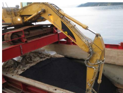
Figure 13: The cover should be removed gradually to avoid loss of heat (Photo: Bjørn Hoven)
