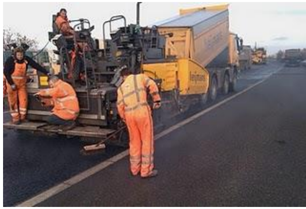
Figure 8: Paving Self-healing Porous Asphalt on the A58 near Vlissingen and the first healing action after three years
