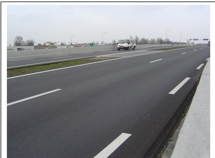
Figure 11: Example application of two layer porous asphalt (Twinlay M) on a provincial road: The N302 at Harderwijk (including the BrainJoint as a Jointless Joint)
