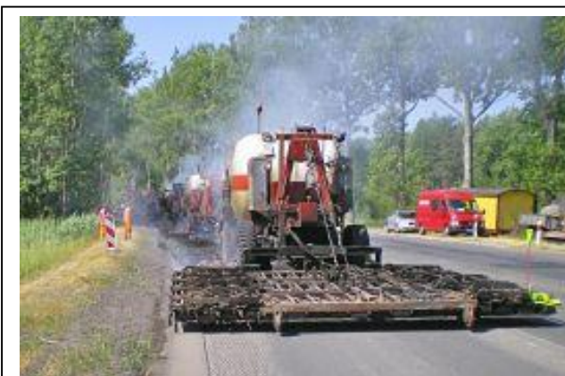
Figure 3: Conventional heating method: Bleu smoke
