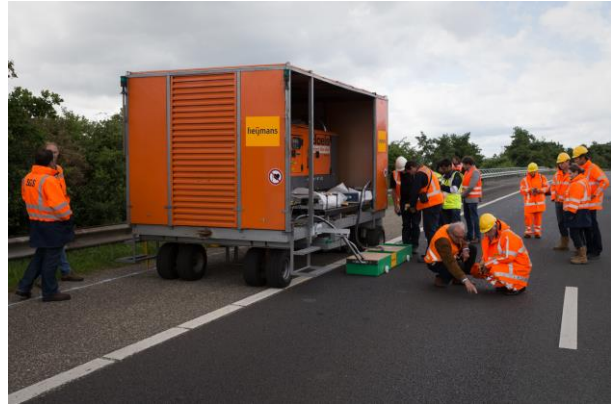
Figure 8: Paving Self-healing Porous Asphalt on the A58 near Vlissingen and the first healing action after three years
