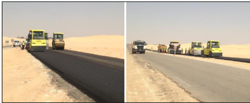
Figure 8: Road construction at Ouargla with Bitumen In-block on April 13 th , 2015.
