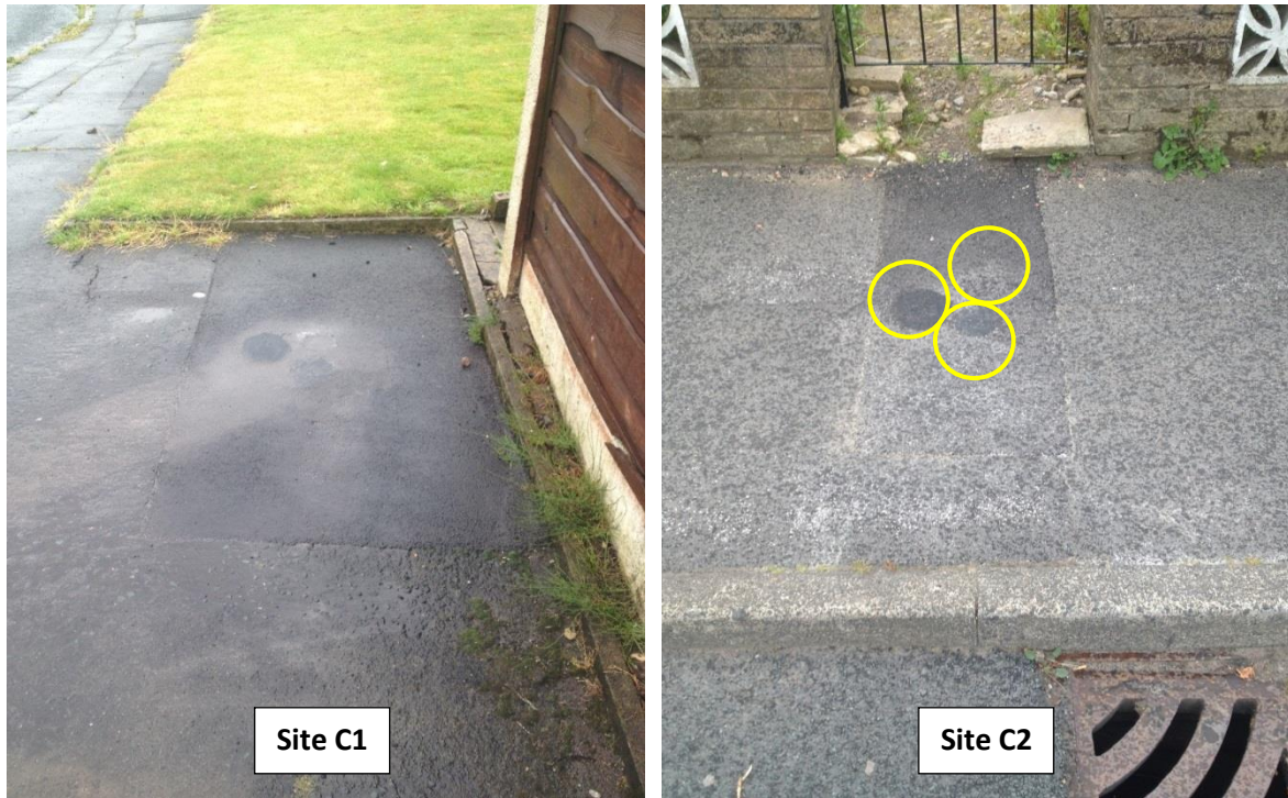
Figure 1: Location of three cores taken by Lab A, Lab B and Lab C from site C1 and C2
