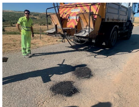
Photograph 14: Cold patch truck Avila Provincial Council
