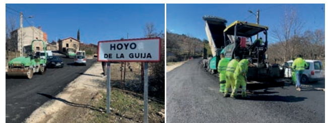
Photograph 18: Sequence of the spreading and compacting works
