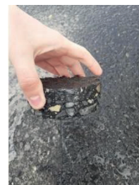
Photo 21: Quality control by extraction of cores in the finished layer
