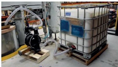
Photograph 13. BIOROAD WARM MIX additive in plant
