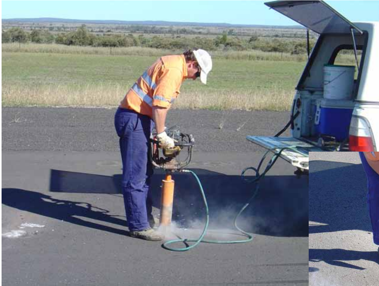
Dry coring before treatment
