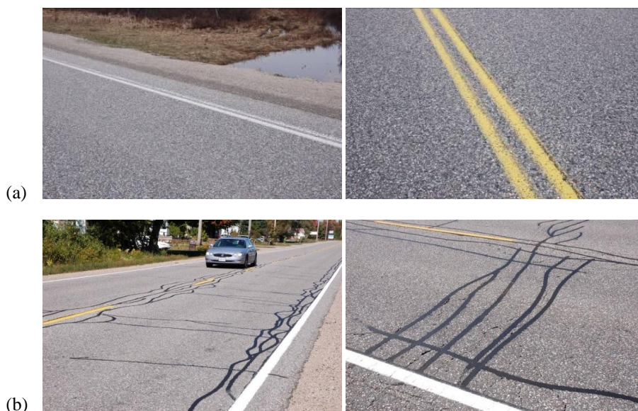
FIGURE 1 – Performance variation for bitumens of nearly identical Superpave grades but different rheological type ((a) sol-type versus (b) gel-type) [15].
