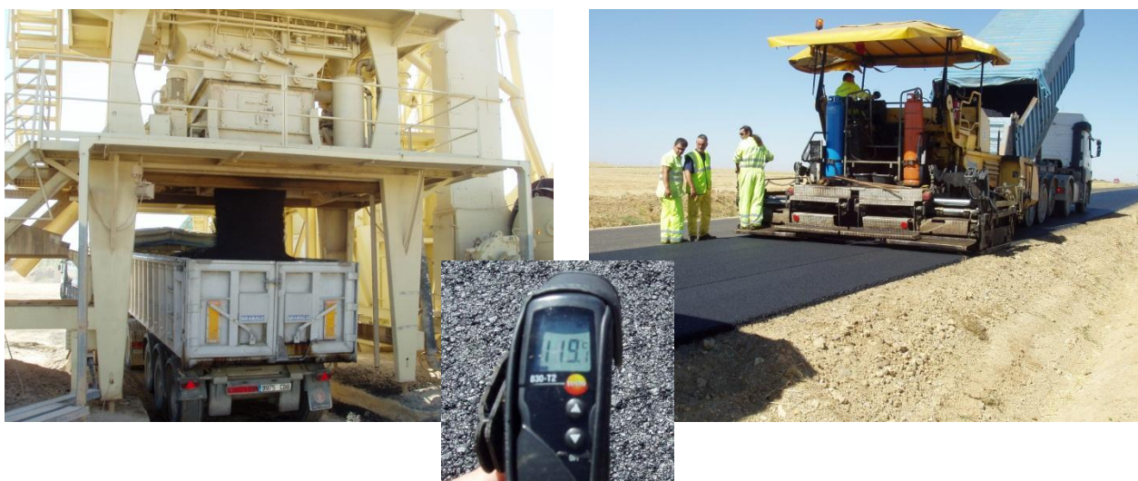
Picture 2: Manufacture and laying of the WMA.
