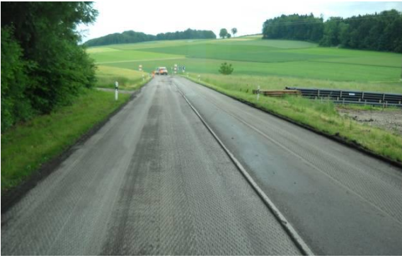
Figure 11: Underground after milling and before laying of the asphalt
