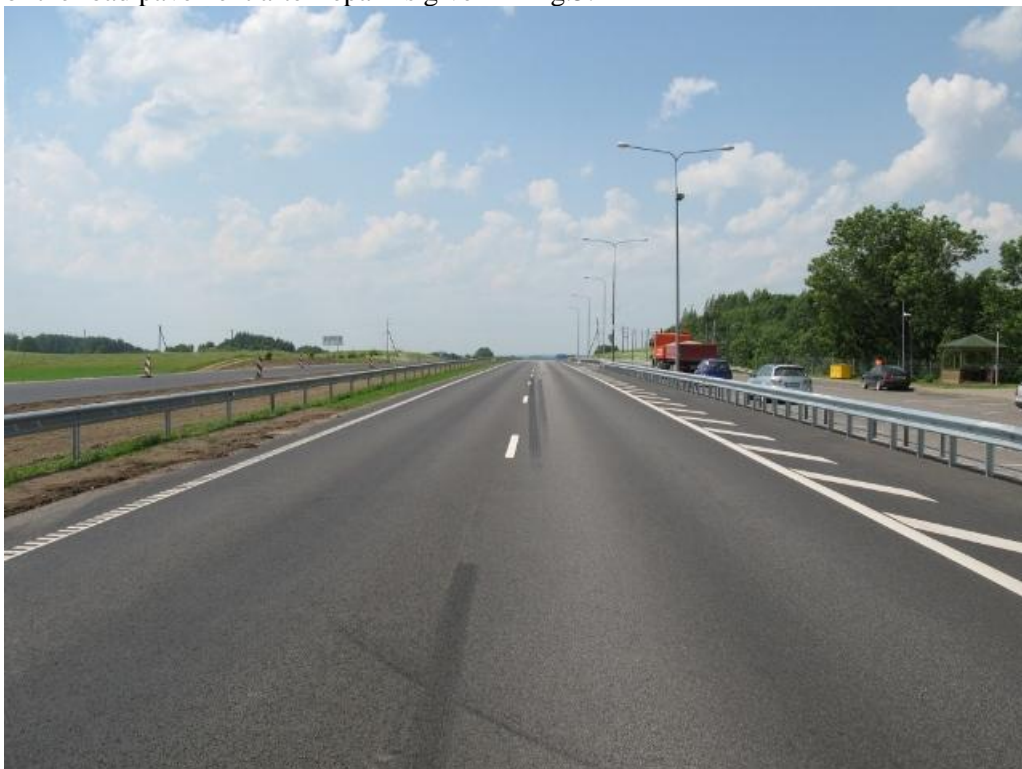
Figure 5. Road A1 Vilnius-Kaunas-Klaipeda (216,95-220,3) km pavement structure after repair
