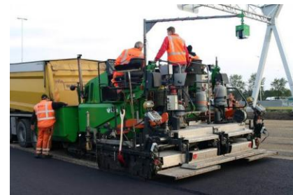
Figure 1: Linescanner behind paver
