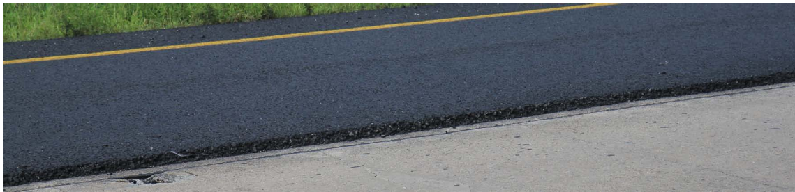
Virginia DoT: SMA over PCC, produced using Warm Mix Asphalt techniques
