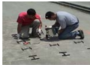
NCAT Strain gauge installation#
