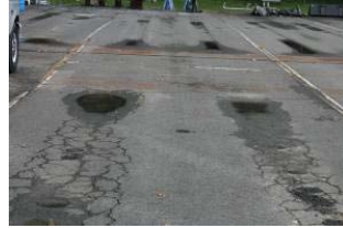
TFHRC Front: Fatigue tests, Back: Rutting tests*
