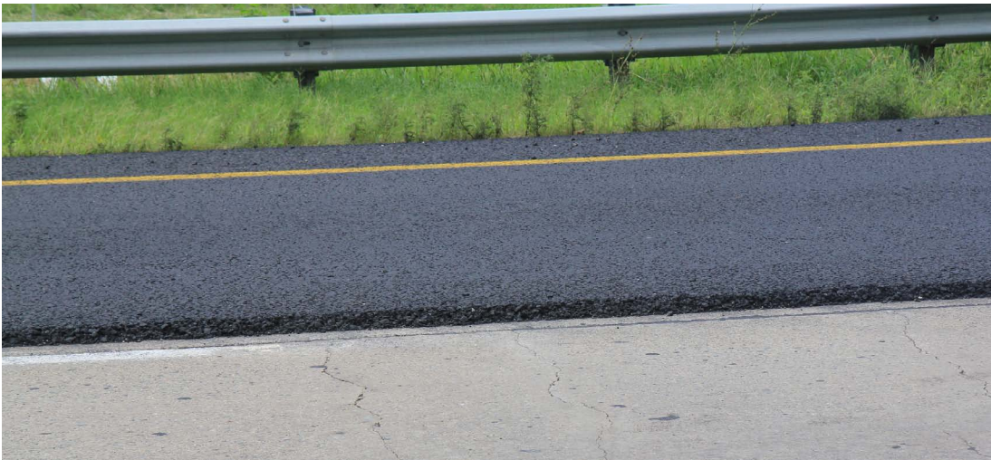
Stone Mastic Asphalt in Virginia to overlay cracked concrete pavements
