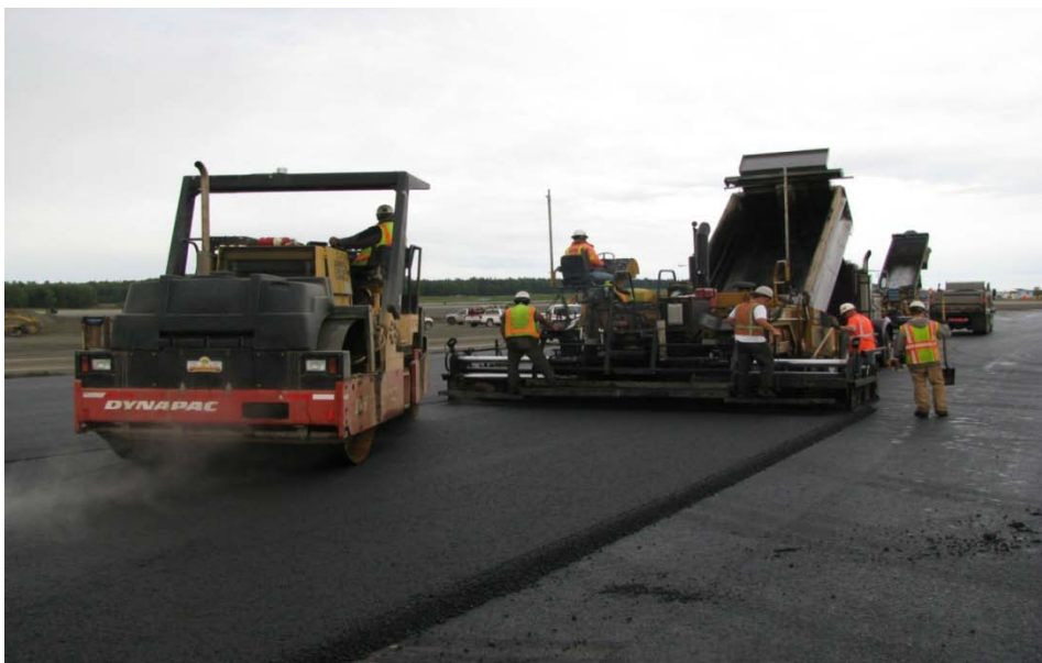
Placement of WMA at Anchorage International Airport
