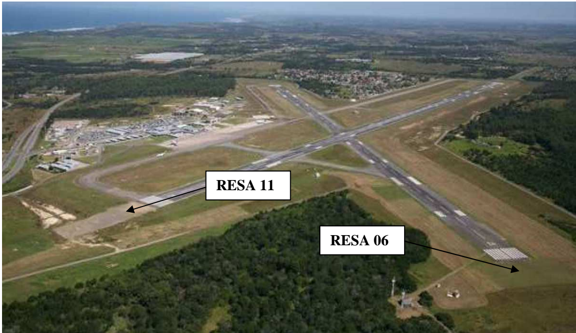
Figure 26 : RESA 11 Before Upgrade
