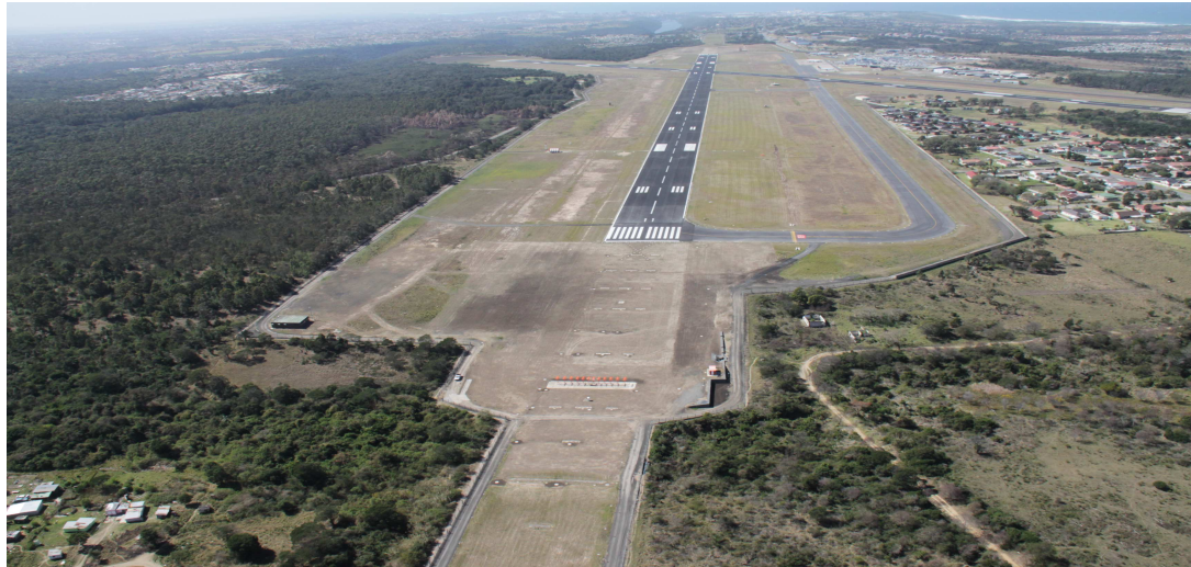
Figure 29 : RESA 29 After Upgrade
