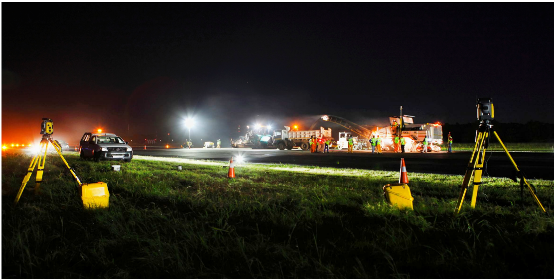
Figure 20 : 3D Milling
