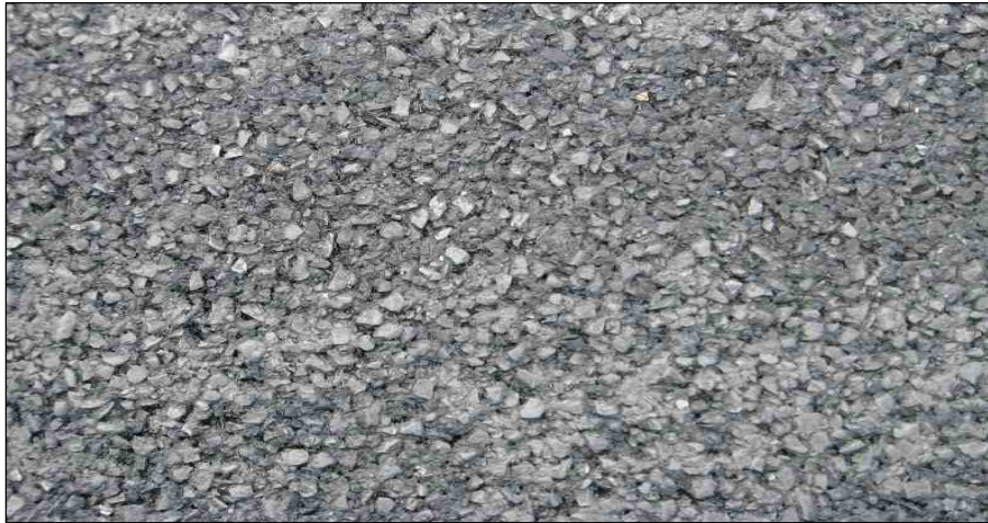
Figure 19(b) : UTFc Friction Layer Trial (Many Surface and Interconnected Voids)
