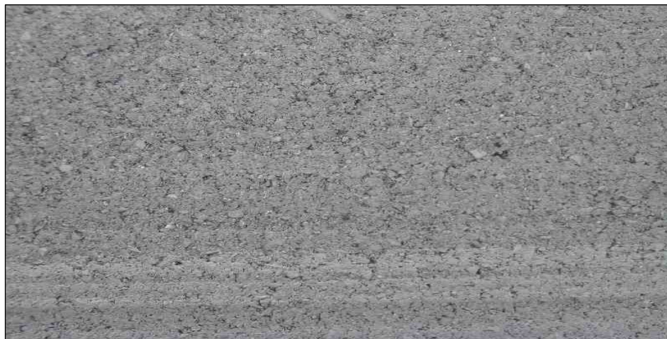
Figure : 19(a) Existing Asphalt (AC) Surfacing With Very Little Surface Voids
