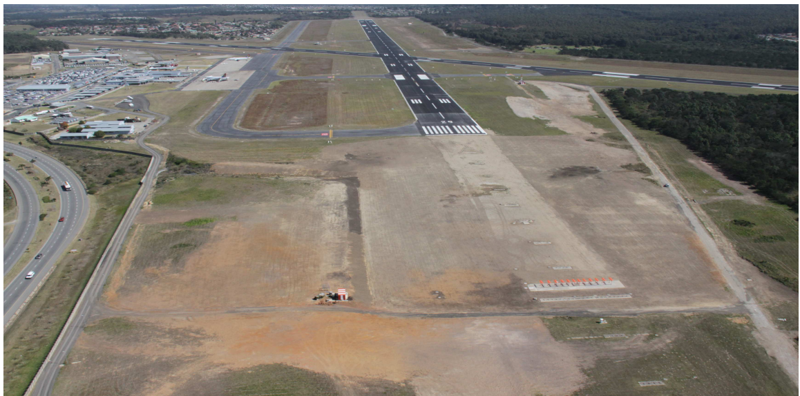
Figure 27 : RESA 11 After Upgrade
