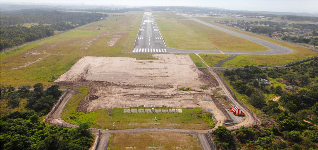
Figure 28 : RESA 29 During Construction
