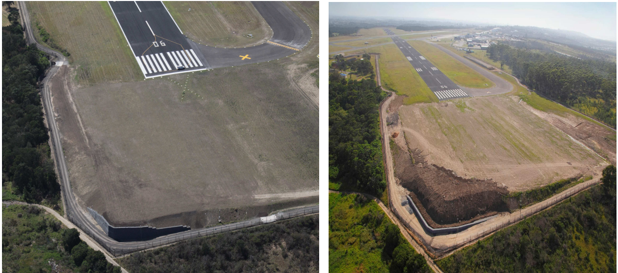
Figure 24 : Retaining Wall at RESA 24
