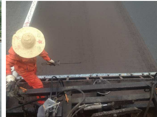
September 2013: Ninglian expressway low noise fiber micro surfacing
