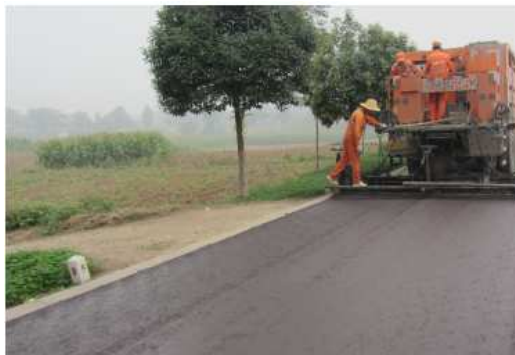
Laying of Fiber Micro Surfacing
