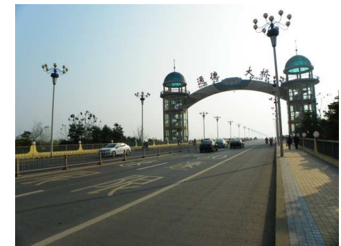
October 2013 Sichuan Suining Tongde Bridge Fiber micro surfacing
