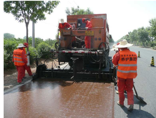
June 2013 Focus Beijing Pinggu Xiayu Road Cape Seal with Fiber micro surfacing
