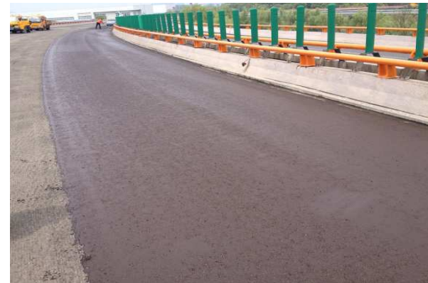
March 2014 - Wuxi SHENGTONG Nanjing Airport Expressway Fiber micro surfacing
