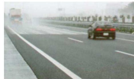
Porous Asphalt Pavement
