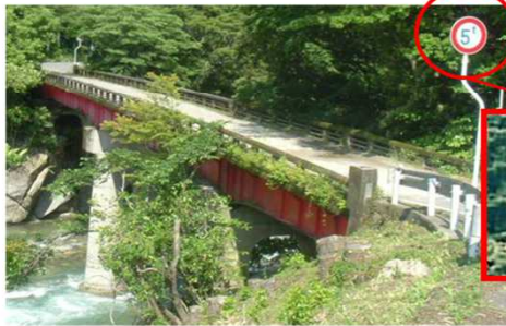
Load Limitation (25t to 5t) caused by severe distress of concrete slab Kamihouri-bridge(Miyazaki)
