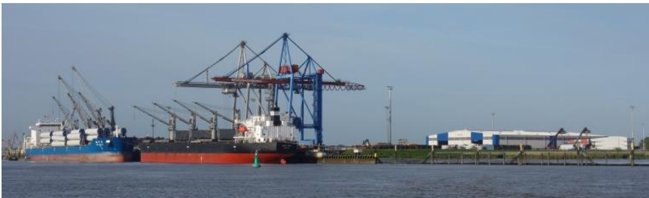
Figure 8: Overview from the upstream face on the Niedersachsenkai with two handysize bulker at the berth
