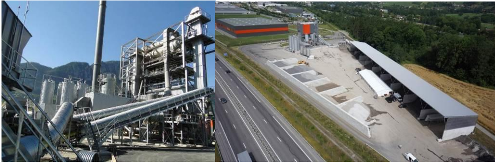
Figure 1: The mixing plant and an aerial view of the Bonneville site
