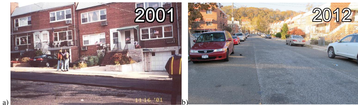
Figure 1. 100% RAP pavement on 75 th street in NYC, Woodhaven at construction (2001) and in 2012 [5]
