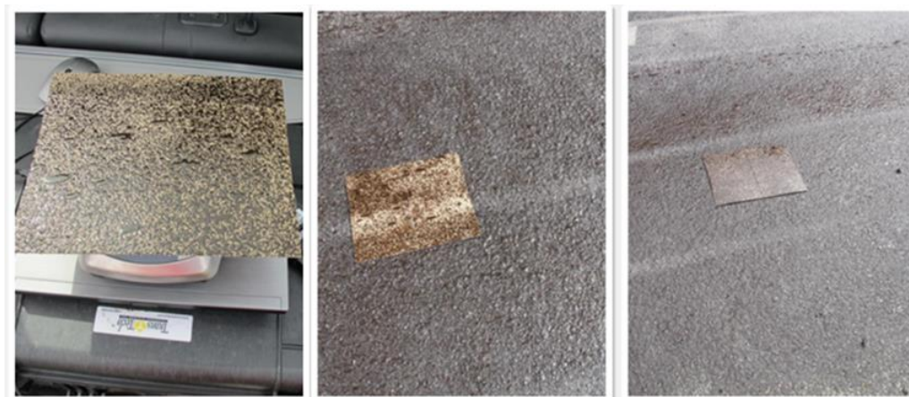
Figure 5: Pads used for measuring tack coat (emulsion) application rates.
