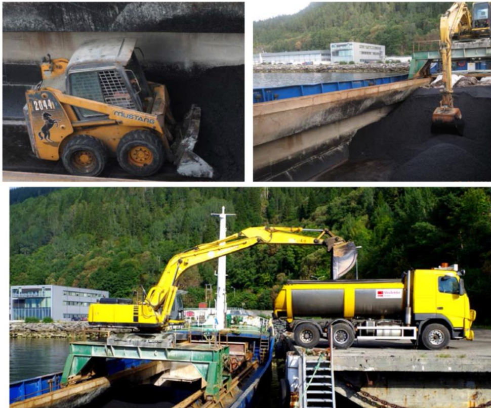
Figure 14: Examples from guidelines of asphalt transport by boat: Cold asphalt from bottom and edges of the loading room must not be loaded on one single truck. And the truck should be perpendicular to the side of the boat during unloading to prevent segregation.
