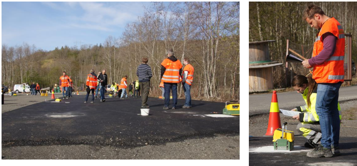
Figure 16: Asphalt inspector gathering; here comparison of asphalt density gauges.
