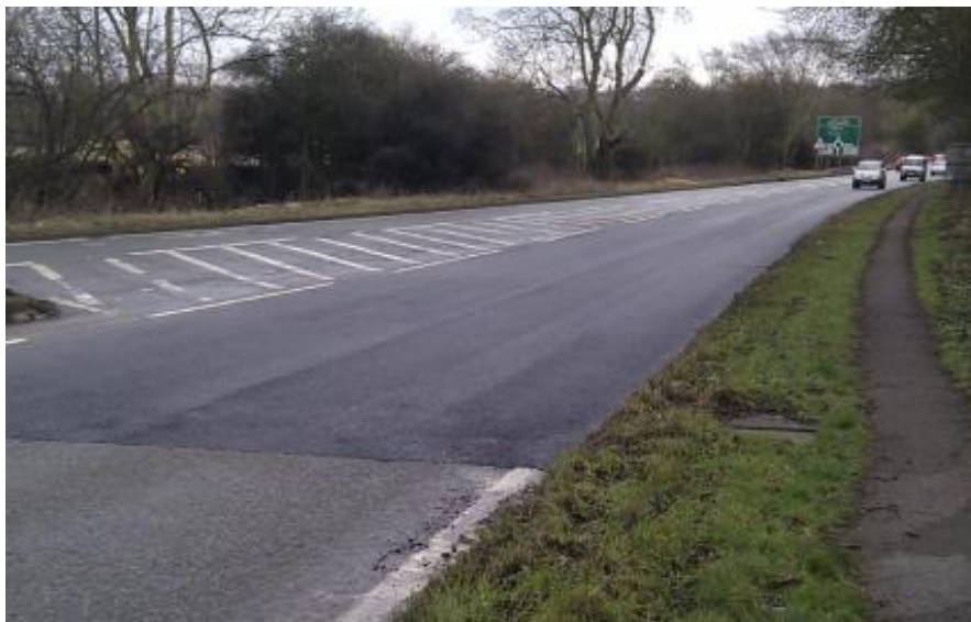
Figure 1: Location of the demonstration site within the A5 Grendon to Mancetter maintenance scheme
