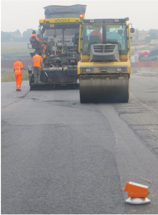
Figure 7 – Trial 1, laying compaction, and density control
