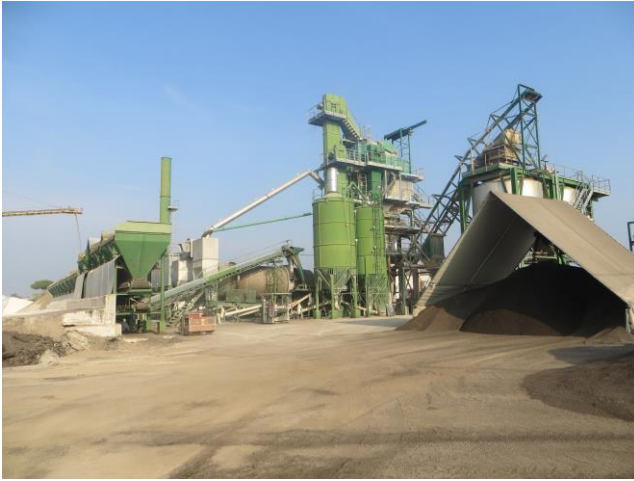
Figure 2 – Plant 1, batch plant with double line RA feeding
