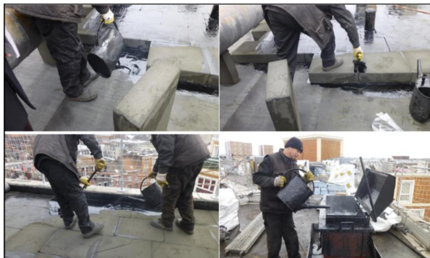
Figure 4: No smoke was emitted during bonding of foam glass with Bitumen B at 160°C.
