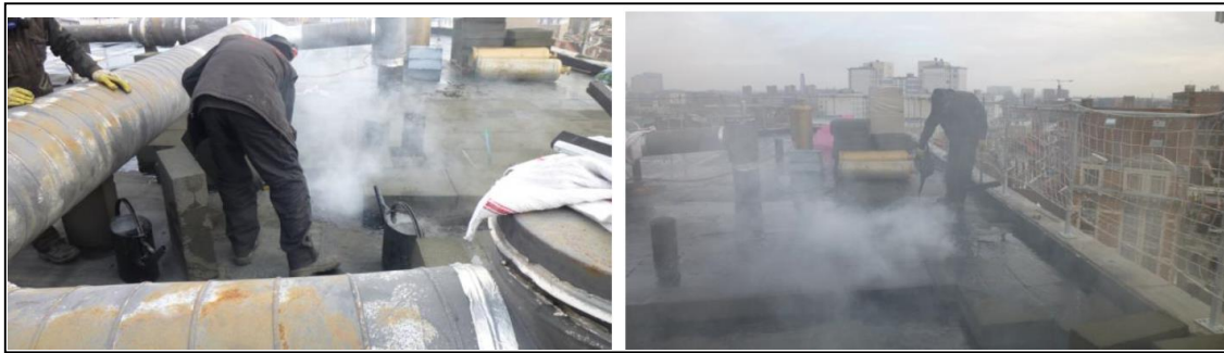
Figure 3: Bonding of foam glass blocks with B ox1 : significant smoke emissions were noted.
