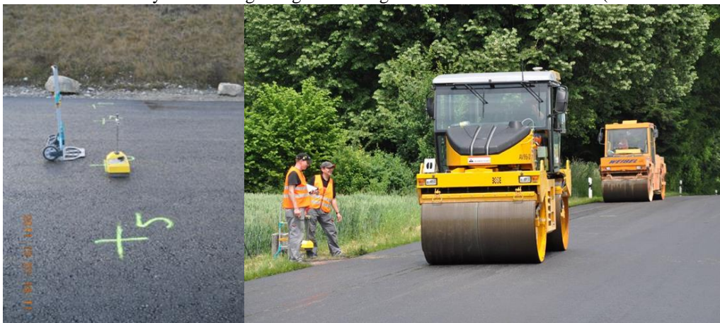
Figure 2: Density measurements are done after each roller pass (right) using a nuclear density gauge (left).
