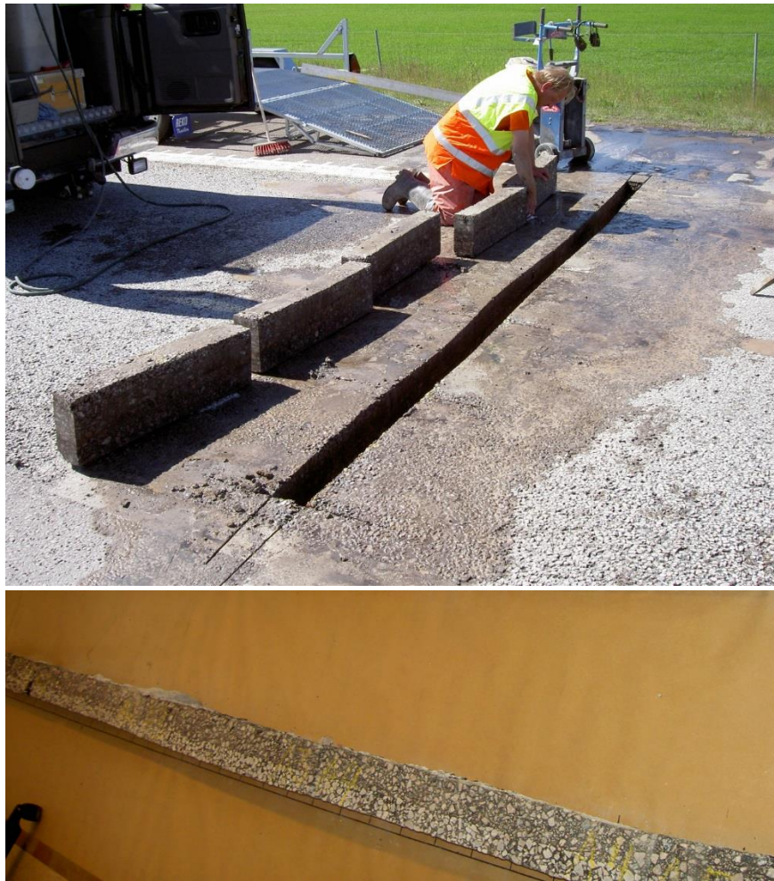
Figure 4: Pavement profile and extracted asphalt concrete beam
